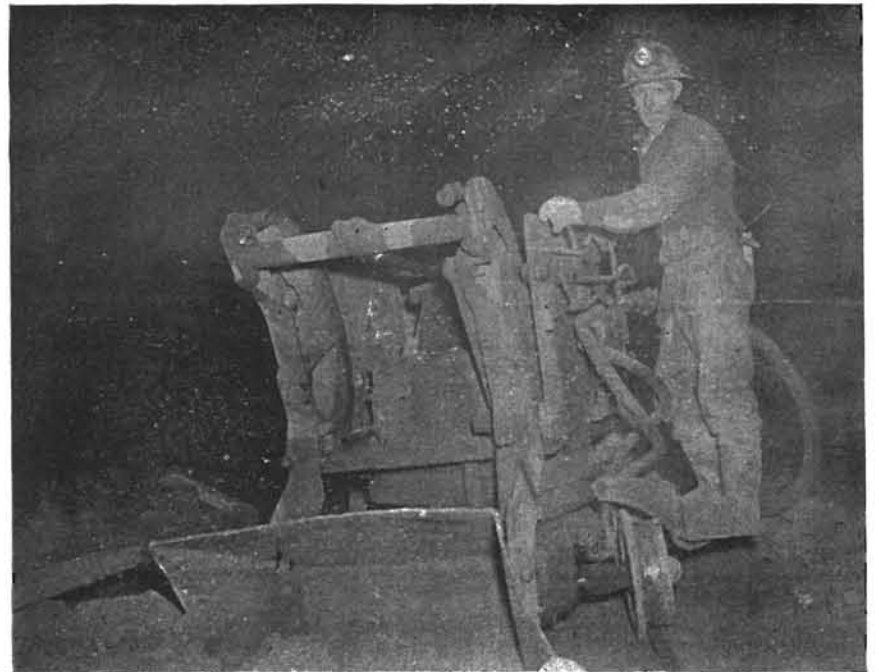
John Karvonen, operating an air shovel-loader while tramming in a drift
