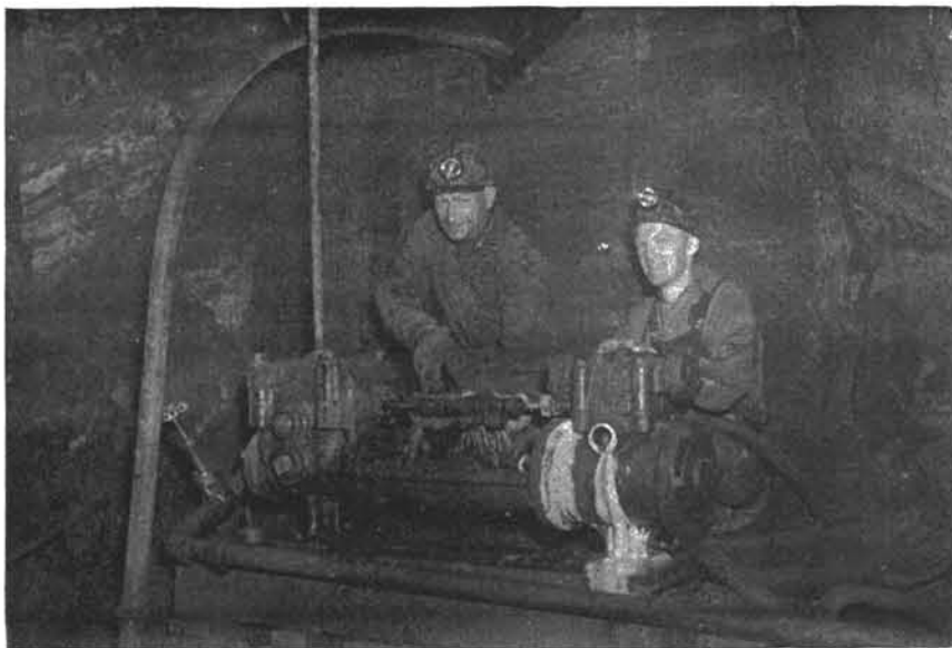
Repairing and operating an underground pump. Allouez No. 3 Shaft House.
