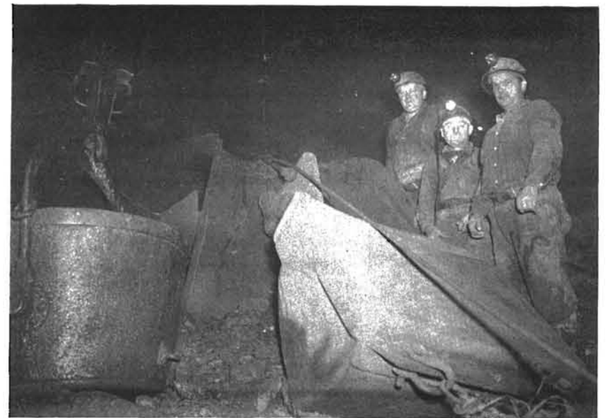
Shaft Sinking Crew, showing bucket, scraper slide and scraper. Erick Harju, Antti Palkki, Henry Hirvonen.
