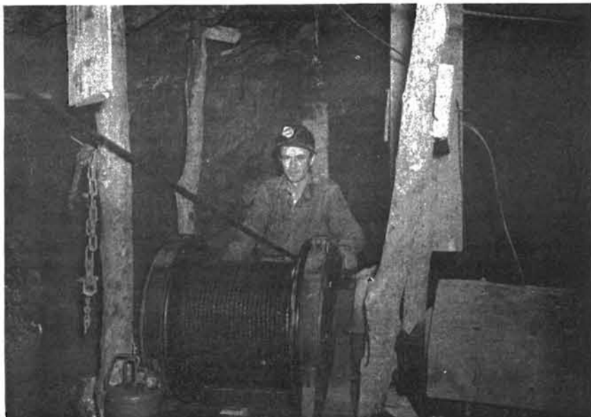
Shaft Sinking Electric Hoist. Roy Bolf, Operator.
