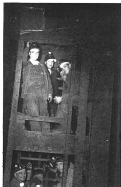
No. 4 shaft, Ahmeek. Showing transmitter mounted in metal case on top of cage. Pull switch is mounted in upper deck.
