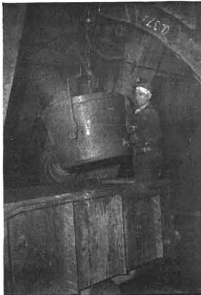
John Panijan, about to dump shaft sinking rock into tram car at bottom level.
