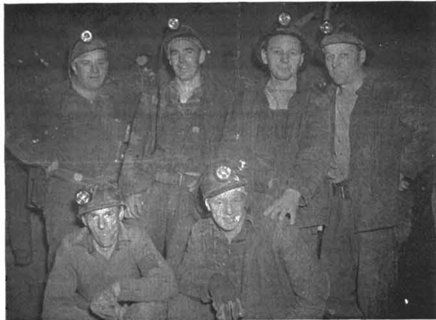
A Shaft Sinking Crew Standing: "Bill" Tapio, "Jim" Whitford, Frank Leidl, Louis Sandretto. Kneeling: Jos. Sitar, "Billy" Gregurich.
