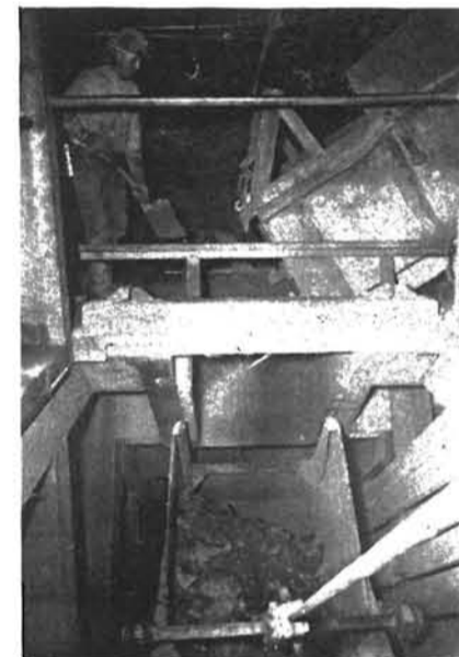
John Kipina, dumping car of rock into skip underground.
