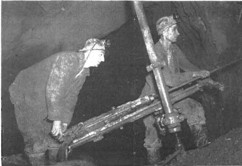
Rigged up and drilling for a chute hole. John Massoglia and John Pastor.
